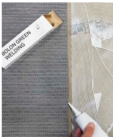
7. Stryk Bolon Green Welding utmed mattans kant.
