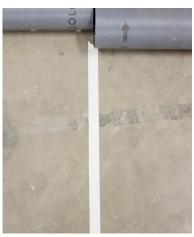
**4.** Roll/fold over the adjoining sheet and put masking tape on the sub-floor along the middle of the joint.
