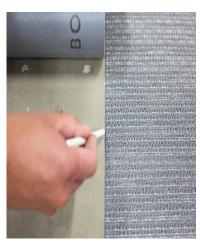
**3.** Roll/fold the first sheet. Mark the position of the joint on the subfloor.
