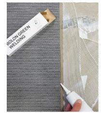
**7.** Add Bolon Green Welding along the cross-section area of the sheet. Avoid overflow on floor covering surface.
