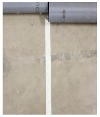
**4.** Roll/fold over the adjoining sheet and put masking tape on the sub-floor along the middle of the joint.
